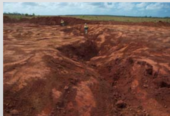
Overburden removal uncovered hidden anomalies, such as this old drainage line
